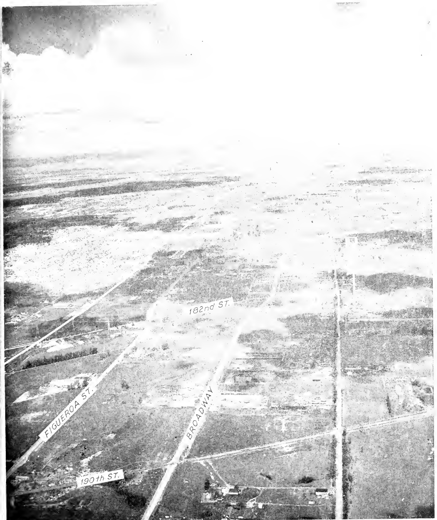
Looking northerly along route of Harbor Freeway showing Los Angeles downtown area, background, right. This portion of alignment was carefully located to clear oil production facilities.
